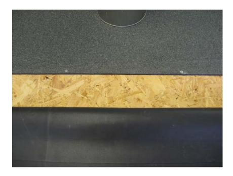
Apply contact adhesive to the back of the membrane and also the deck...
