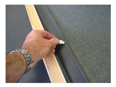
Apply a bead of Water Block sealant underneath the edge of the membrane.
