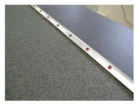
**Important note:** Termination bars have to be cut at angle changes, and not bent around corners. The resulting ends are to be spaced no more than 10mm apart. A patch of Quickseam Formflash is also required to waterproof this area.
