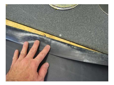
Then create a straight edge on the membrane using a crayon and cut away any excess material along the line.
