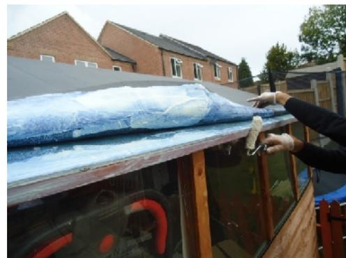
**IMPORTANT.** There are various shed designs along the water run off edge as shown above. We recommend that a thin layer of adhesive is applied to the back of the rubber membrane also, and allowed to go semi dry. (It will start to go clear looking). We also recommend a thin layer of adhesive to any part of the timber area that you would like the rubber membrane to adhere to. The
