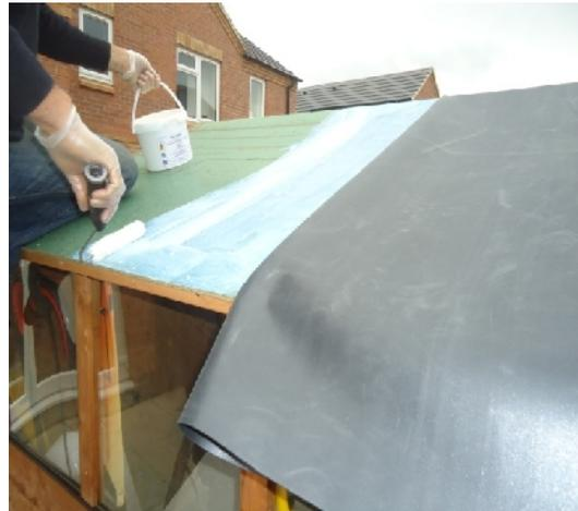
**STEP 4.** Trim off any excess rubber sheet around the edges, leaving approx. 50mm overhang
