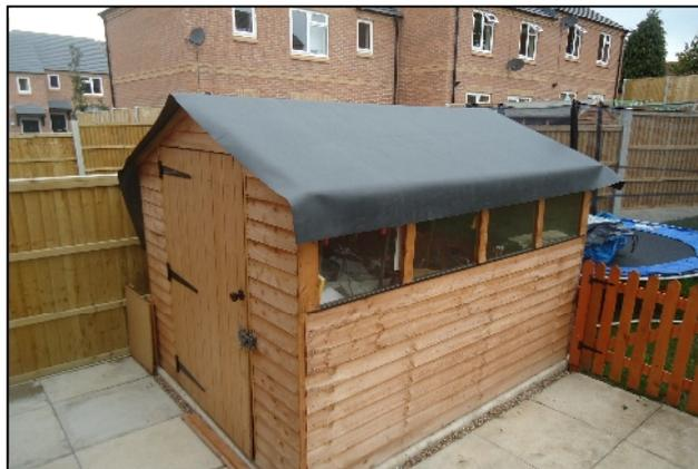
**Step 3.** Fold half the membrane back on itself and apply water based adhesive to the roof deck using the mini roller enclosed. Repeat the process on the other half. A pair of protective latex gloves are enclosed for cleaner application. Broom over surface of membrane to ease out any creases or bubbles.
