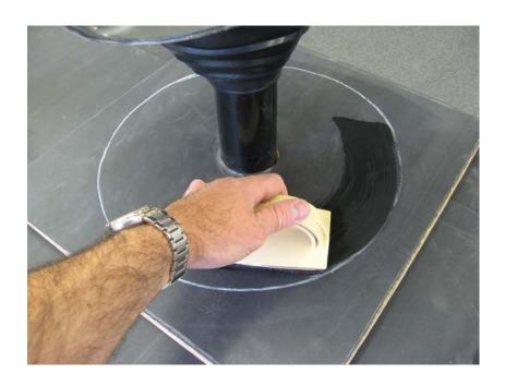
Place the boot back into position on the deck and peel away the backing paper from underneath.
