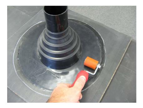
Pull the top of the boot around the neck of the pipe to allow Lap Sealant to be applied.
