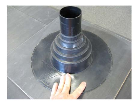
With the crayon, mark out the area to be primed approx. 10mm from the base of the boot.
