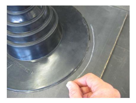
Lift the boot upwards to apply the Quickprime plus onto the deck.
