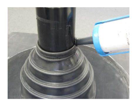
Then close up the top of the boot to cover the Lap Sealant...
