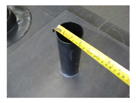
and cut out the same diameter within the pipe boot flange...
