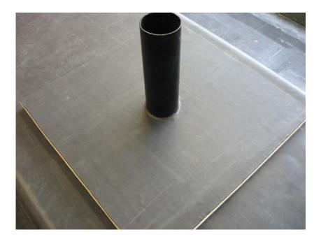
It doesn't matter what diameter of pipe you are waterproofing as the procedure for this detail is the same. There are 3 pieces of Quickseam Formflash needed to complete this detail, two of which are the same size for the base area, and one to wrap around the pipe.
