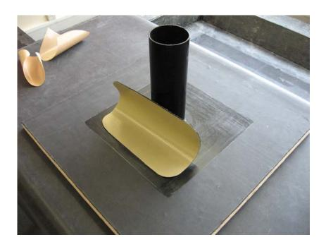
On the reverse of the tape, mark and cut out a bell shape as shown below, 25mm smaller than the dimensions of the pipe. This will create a small upstand on the pipe.
