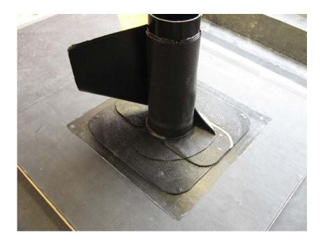
Apply the Quickprime Plus and once it is dry, attach the overlap to the pipe, and bring the rest of the Quickseam Formflash onto the deck. Use the rollers as normal.
