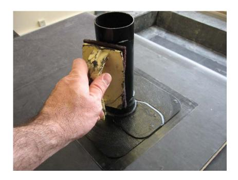
Apply Quickseam Formflash and wrap around the pipe as shown below:-
