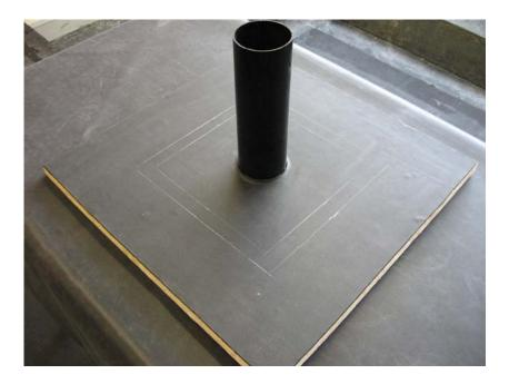
Prime the 95mm area around the pipe, and also part way up, and wait until dry.
