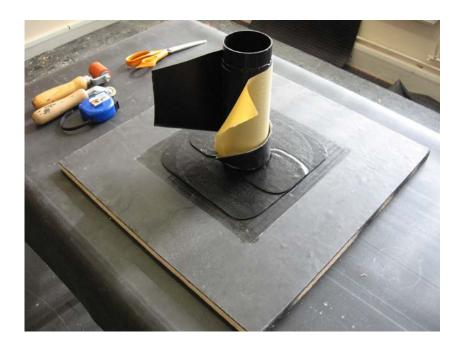
Quickprime Plus needs to be applied where the overlap will attach, so start to lay the Quickseam Formflash onto the deck, but only enough (approx. 125mm) for the Quickprime Plus to be applied.
