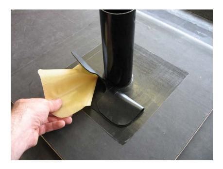
...and lay the Quickseam Formflash around the pipe, keeping the edges in line with the 75mm markings.
