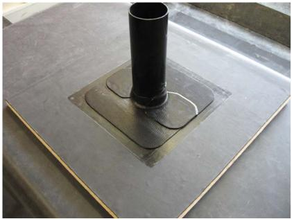
The final piece of Quickseam Formflash wraps around the pipe, and is then laid onto the deck by 50mm. The size of Quickseam Formflash needed = circumference of the pipe + 100mm for the overlap. E.g., a pipe with a 320mm circumference will require a 420mm piece of Quickseam Formflash.
