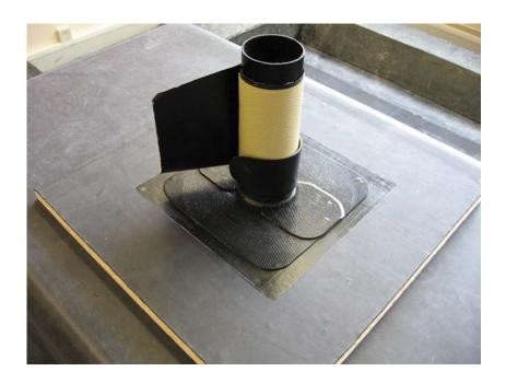
With the yellow plastic backing still attached, "roll" the Quickseam Formflash down the pipe towards the base, then peel the first few inches of the plastic backing away.
