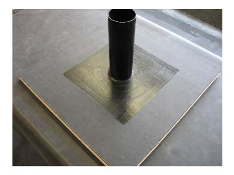
Round the corners off the Quickseam Formflash, and mate onto the deck in line with the 75mm markings.
