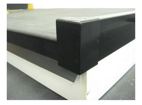
Finish off with the corner end caps. These are attached with a small amount of superglue.
