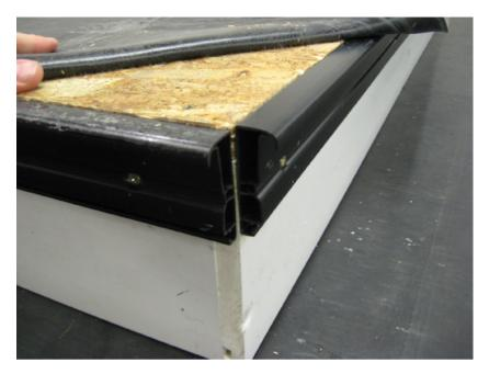
With the membrane hanging over the edges, secure the drip plates. The excess that remains between the two edges can now be covered by a modified external corner piece of Permaroof trim. Remove the excesses as shown below...
