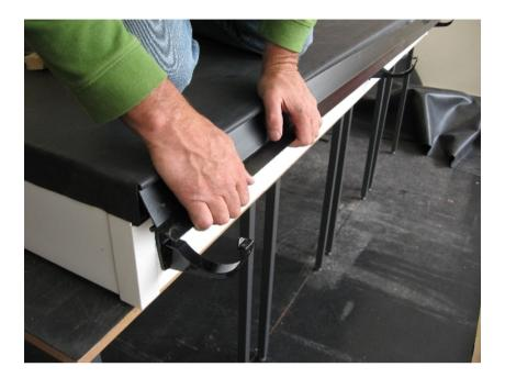
... then the drip plate can be tapped firmly into place until it clips in securely. The use of a short piece of batten and a hammer or even a rubber mallet will ensure that the drip plate will not be damaged during fitting. Do not strike the drip plate directly.
