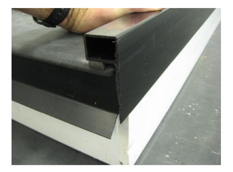
For corner pieces, apply a small amount of Permaroof Bond 'n' Seal on the inside of the corner, and offer into place. Alternatively, pre-drill a small hole in the corner piece and attach with a poly top pin.
