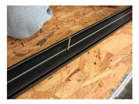
Make sure that the top of the backplate is flush with the surface of the roof deck, and then secure with the fixings.
