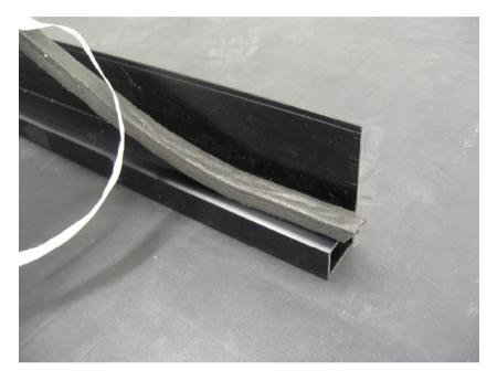
Trim the membrane so that maximum 50mm overhangs the perimeter edges. Starting at one corner, fold the small excess of membrane away...
