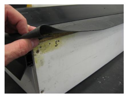
...offer the trim into place and fix securely. There are pre-drilled 5mm slots every 300mm down the length of the trim for easy fitting.
