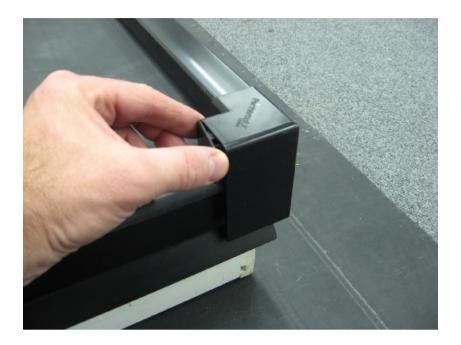
When joining lengths of Permaroof trim, cap the ends off by applying end caps, and offering into place.
