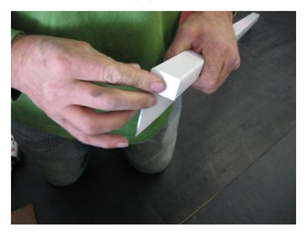
Attach the trim as already described, butting the two lengths together, with a bead of Permaroof Bond 'n' Seal or foam tape in between.
