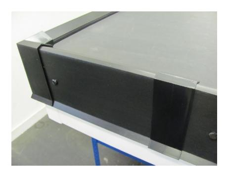
The roof is now ready to receive the Permaroof Plus gutter edge trim drip plate.
