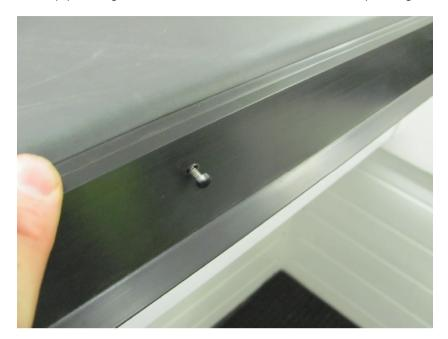
Seal the top edge with an additional bead of Permaroof Bond  $^{\prime}$ n $^{\prime}$  Seal and remove excess sealant.
