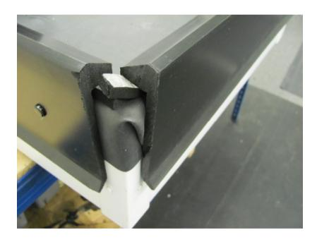
Attach a prefabricated external corner piece and secure with either Permaroof Bond 'n' Seal or Superglue.
