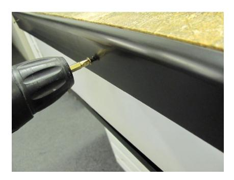
Once the membrane is applied to the roof deck as described elsewhere in this manual, application of the Permaroof Plus trim system can be finished.
