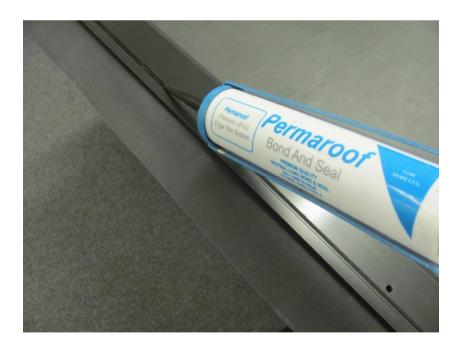
Offer up the drip plate and secure with BP40 polytop pins. Take care not to locate the top of the drip plate higher than roof deck level as this will cause ponding on the roof.
