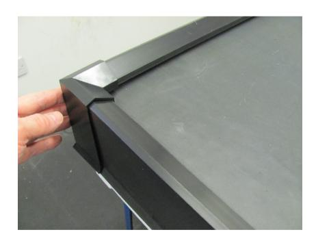
For corner pieces terminating around onto a gutter edge, use a small pre-cut piece of kerb trim and secure with either the sealant or the glue inside the external corner. This will close up the void created by the external corner termination.
