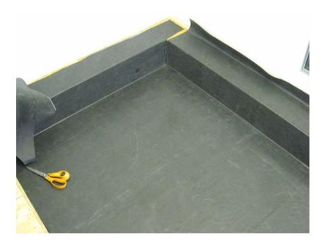
A Quickseam Formflash patch is the finishing detail for this corner...
