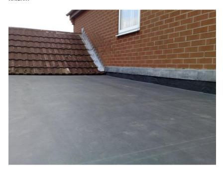
...and also metal wall trim. If attaching metal wall trim into a wall chase, use Permaroof Bond 'n' Seal to waterproof the top edge of this trim, and mechanically fix the trim to the perimeter wall with tech fixings.
