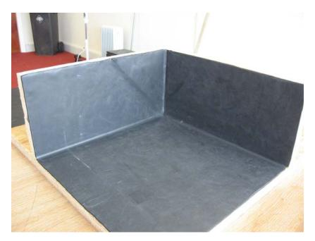
The following pictures show the internal corner being formed on top of a parapet wall.
