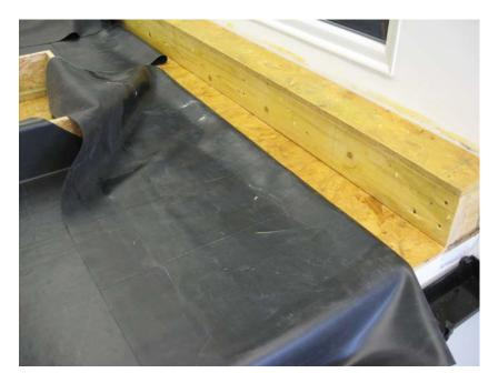
When applying the contact adhesive, all areas have to be clean and dry. The adhesive can be applied with either a small 4" roller or similar size paintbrush. Care needs to be taken when using contact adhesive. Adhesive spillages can swell the membrane, so it is worth keeping the adhesive and rollers away from the roof membrane. An offcut of EPDM is ideal as a base for the adhesive tin.
