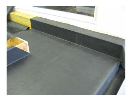
When one wall is adhered, start to adhere the adjoining wall. An excess of material will collect in the corner, which needs to be tidied up and secured. This excess is commonly known as the "pig's ear".
