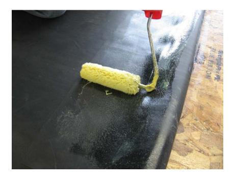
Once the adhesive is tacky, offer up the membrane by rolling it into the angle change and then up the wall. This method prevents any tenting of the membrane at the angle change.
