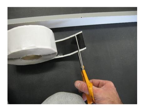
$50 \text{mm} \times 25 \text{mm}$  of tape is adequate for each fixing. The fixing points are evenly distributed and are generally 600 mm apart. Apply the tape to the underside as shown, and peel off the backing paper.
