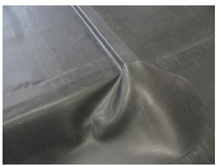
At the gutter edge, excess membrane needs to be trimmed off. Mark the membrane with the blunt edge of the scissors against the gutter and cut away the excess. The remaining membrane will fall naturally into the gutter at the correct length.
