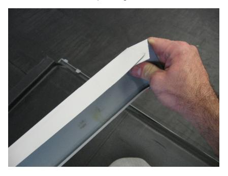
Butyl sealing tape needs to be applied to the underside of the trims at the fixing points to waterproof the fixing penetration.
