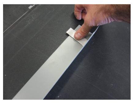
Tech screws are used for attaching the trim. These screws cut through the trim, the butyl sealing tape and into the batten with no pilot holes required. Offer the trim to the desired position on the edge, and fix with a cordless screwdriver.
