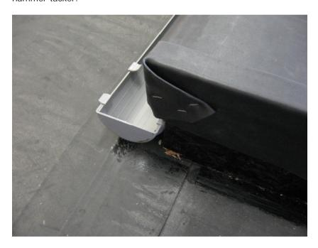
Use the tin snips to cut the trims to size. For corner details, cut the top edge and also a V-shape in the trough at the bottom edge of the trim also.
