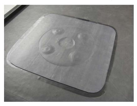
Remove the SA flashing covering the outlet by cutting a hole around its diameter. Take care not to cut into the drain outlet itself.
