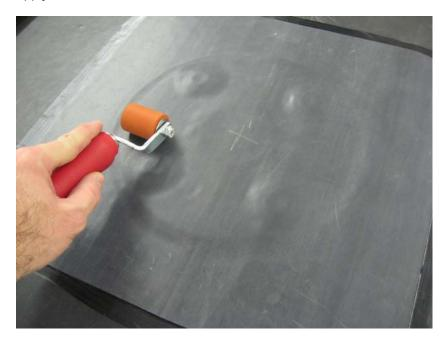
Note that Quickprime plus should be visible around the edge of the flashing.
