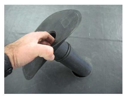
Mechanically fix the outlet to the roof deck using V-plates and All-purpose fasteners.
