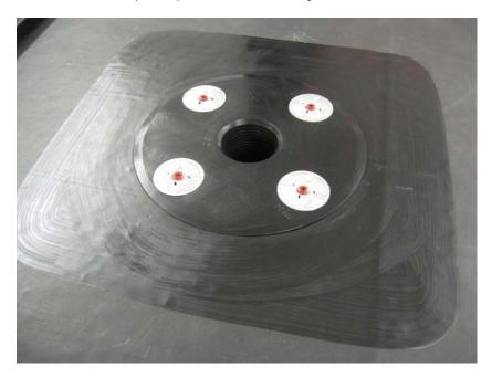
Prepare a piece of SA flashing minimum 75mm larger than the drain outlet diameter and apply to the primed area.
