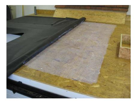
Note that the water-based bonding adhesive does not go right up to the perimeter edge of the roof deck, but instead terminates 100-150mm away. This area is where the yellow contact adhesive will be applied later. The water-based bonding adhesive can take up to a few hours to grab the membrane completely, but the use of the yellow contact adhesive around the perimeter edges secures the sheet in place during this period.
