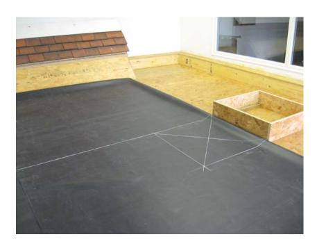
Cut a straight line from the nearest edge of the membrane to one corner, then cut the X mark.
