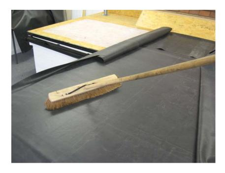
Roll back the other half of the membrane up to the already applied adhesive and repeat the procedure.
