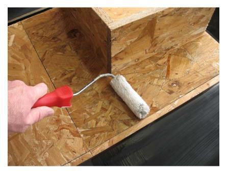
Once the contact adhesive is tacky, offer the membrane to base of the upstand, pushing right into the angle change to eliminate any tenting.
