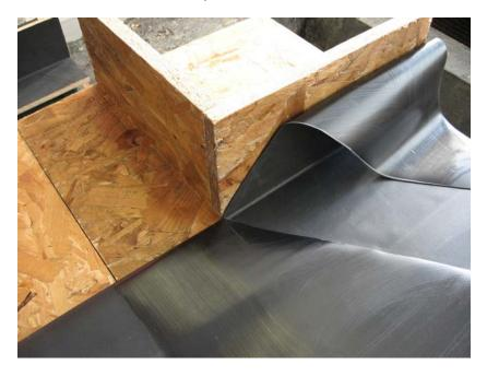
The rest of the membrane can now continue around the corner, and be adhered in place.
