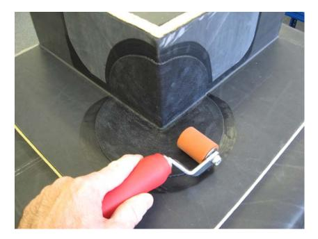
An example of a skylight installation using SA flashing and Quickseam corner flashing.
