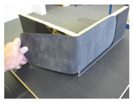
The final waterproofing detail requires a piece of Quickseam cover flashing at the corner at the angle change.
