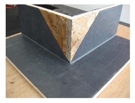
This area now needs to be waterproofed, and this is done with SA Flashing, Quickprime Plus and Quickseam Corner Flashing.
