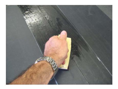
Wait for the Quickprime Plus to go tacky. This is especially important, as the tape will not adhere to it if it is in a wet state. Use the "pushed finger" test, and if the finger moves through the Quickprime Plus or strings in any way (as shown below), it is NOT ready for the tape.
