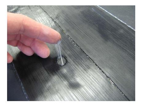
Once the Quickprime Plus is ready, apply the tape to the primed area. Lay the tape parallel to the marked line, keeping the tape taut to prevent air bubbles being caught underneath it. If you run out of tape, overlap the last 50mm with a new roll, but don't forget to apply Quickprime Plus on top. Continue to lay the tape. Once the tape is laid, remember to be overlay the joint with a 150mm x 229mm patch of Quickseam Formflash.
