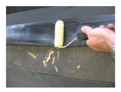
With the membrane adhered to the deck, lay the tape in situ evenly across the join.
