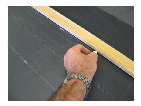
Apply Quickprime Plus with a Quickscrubber pad and handle within the marked area. Apply all the way down the join, avoiding puddles by spreading it out evenly.
