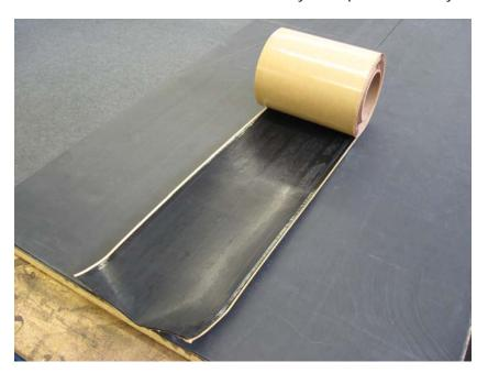
Outline with a crayon where the edges of the tape lie. This gives a guideline for you to apply Quickprime Plus. Make sure that the crayon marks extend beyond the edge of the tape around 10mm each side.
