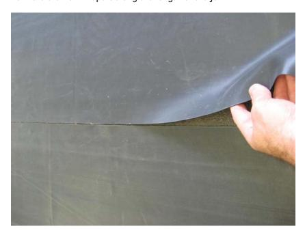
Also make sure that contact adhesive is used on both the back of the membrane and deck surface to secure the edges.
