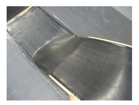
Use the silicon roller to ensure the tape has adhered properly to the membrane, firstly across the joint...
