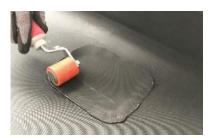
• Smoothen the EasySealant using a piece of (release) liner, plied in V-shape, over the entire seam.
