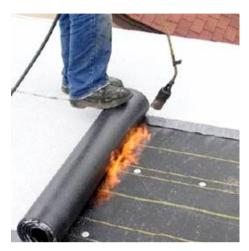
Bituminous roofing felt is a widelyaccepted, (and perhaps the most commonly first-thought-of) option for DIY roofing projects such as shed roofing.
