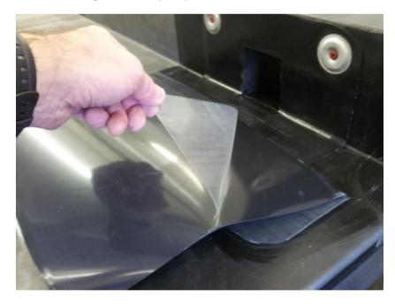
Continue to offer up the SA flashing tight into the angle change and then up the upstand. Apply the silicon roller for total adhesion.
