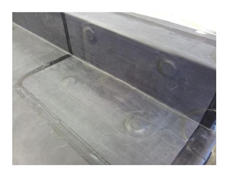
Remove the SA flashing that covers the outlet hole with careful use of a sharp knife. Take care not to cut into the drain outlet itself.
