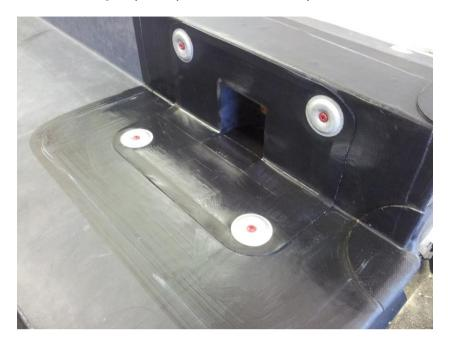
Prepare a piece of SA flashing minimum 75mm larger than the through wall outlet flange. Remove the plastic backing and apply the flashing to the primed area onto the deck, ensuring that the Quickprime Plus is visible all around the flashing edge.
