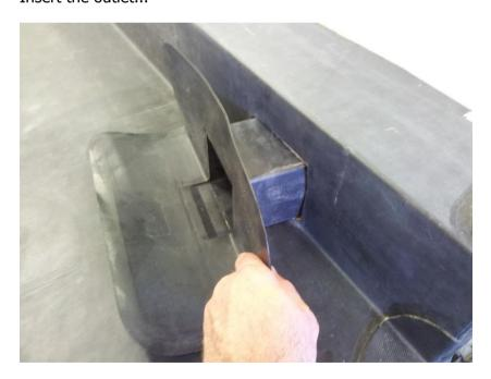
Mechanically fix the outlet to the roof deck and upstand wall using V-plates and All-purpose fasteners.
