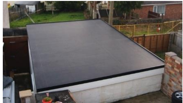
Figure 1: Domestic EPDM flat roof
