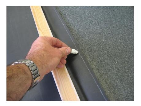
Apply a bead of Firestone Water Block sealant underneath the edge of the membrane.
