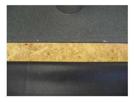
Apply Firestone Bonding Adhesive to the back of the membrane and also the deck...
