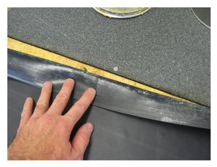
Then create a straight edge on the membrane using a crayon and cut away any excess material along the line.
