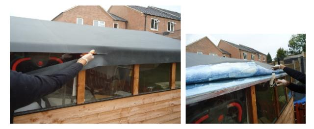
**IMPORTANT.** There are various shed designs along the water run off edge as shown above. We recommend that a thin layer of adhesive is applied to the back of the rubber membrane also, and allowed to go semi dry. (It will start to go clear looking). We also recommend a thin layer of adhesive to any part of the timber area that you would like the rubber membrane to adhere to. The
