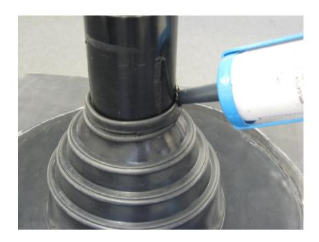
Then close up the top of the boot to cover the sealant...
