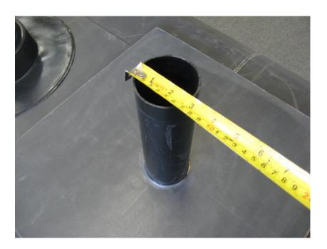
...and cut out the same diameter on the pipe boot flange...
