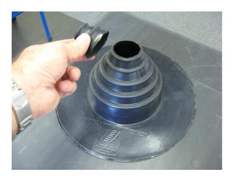
Stretch the boot over the pipe and offer into position onto the deck.
