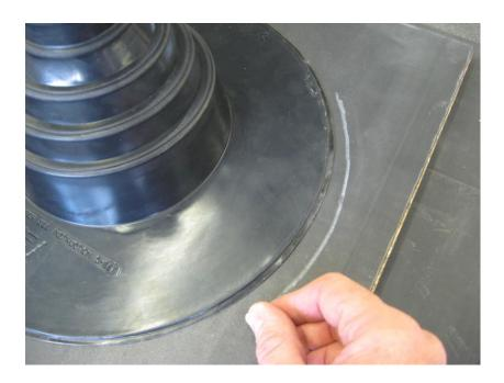
Lift the boot upwards to apply the Quickprime plus onto the deck.
