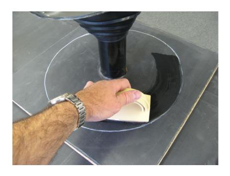
Once the Quickprime Plus becomes tacky, place the boot back into position on the deck and peel away the complete backing paper from underneath.
