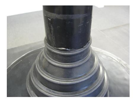
Now apply the clamping ring, and secure into place.
