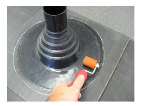
Pull the top of the boot around the neck of the pipe to allow Permaroof Bond and Seal to be applied.
