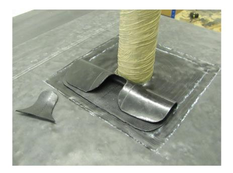
Apply the Quickseam Formflash around the pipe, keeping the edges in line with the 75mm markings.
