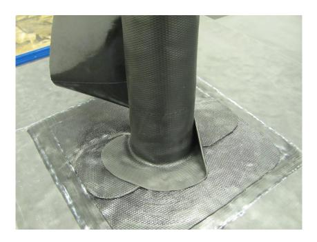
Apply the Quickprime Plus and once it is tacky, attach the overlap to the pipe, and bring the rest of the Quickseam Formflash onto the deck. Use the rollers as normal.
