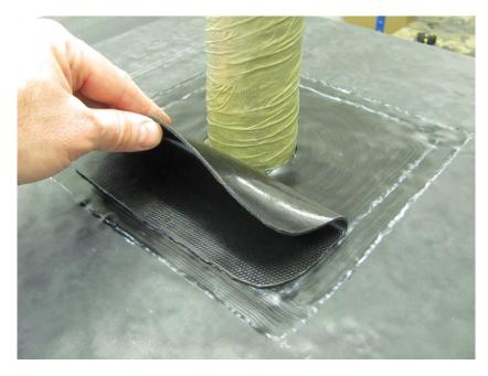
On the reverse of the tape, mark and cut out a bell shape as shown below, 25mm smaller than the dimensions of the pipe. This will create a small upstand on the pipe.
