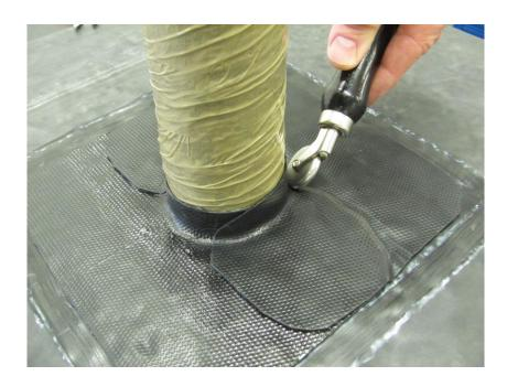
The final piece of Quickseam Formflash wraps around the pipe, and is then laid onto the deck by 50mm. The size of Quickseam Formflash needed = circumference of the pipe + 100mm for the overlap. E.g., a pipe with a 220mm circumference will require a 320mm piece of Quickseam Formflash.
