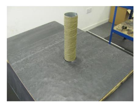
There are 3 pieces of Quickseam Formflash needed to complete this detail, two of which are the same size for the base area, and one to wrap around the pipe. With the crayon, mark out the area to be primed at least 95mm from the pipe. Also mark out 75mm distances as a guideline for applying the Quickseam Formflash.
