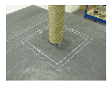
Apply the Quickprime Plus to the outer markings around the pipe, and also approx. 75mm up, and wait until tacky.
