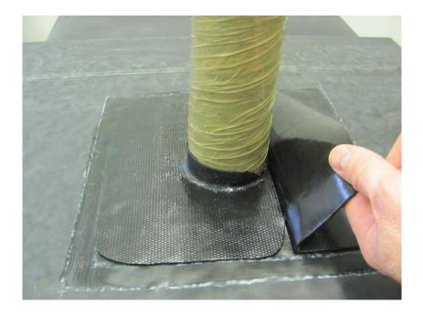
When applying, keep the edges in line with the first piece of Quickseam Formflash and finish with the rollers.
