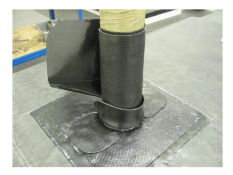
Quickprime Plus needs to be applied where the overlap will attach, so start to lay the Quickseam Formflash onto the deck, but only enough (approx. 125mm) for the Quickprime Plus to be applied.
