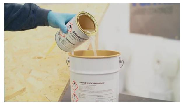
Mix the Permathix into the Permaroof500 (whether accelerated or not) by hand until thoroughly blended. Ensure the Permathix is fully incorporated.
