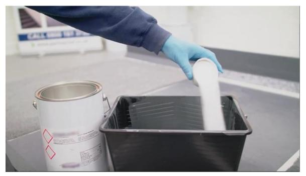
Mix thoroughly at medium speed and ensure the product is well-blended. This plastic bead does not sink to the bottom of the mixed tin or container.
