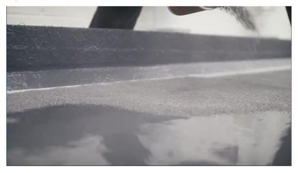
Depending upon the design level required, silica sand, mineral clippings or other suitable anti-slip finishes can be added.
