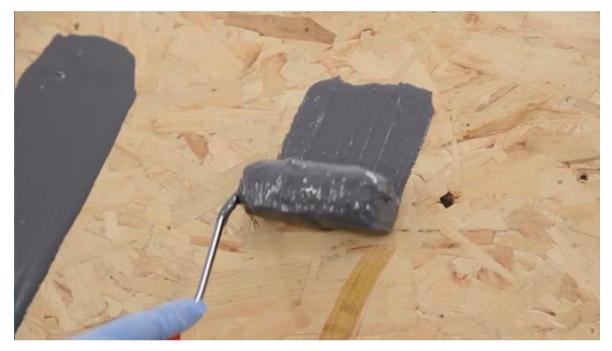
Permathix also allows Permaroof500 to be applied in box gutters with matting in a wet on wet system.
