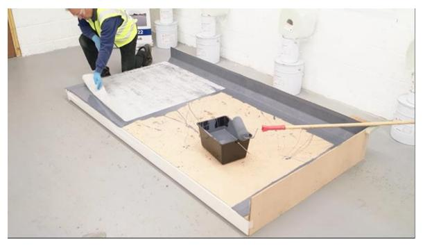
And add another layer of the Permaroof500 liquid EPDM to fully embed the matting before moving to the next section.
