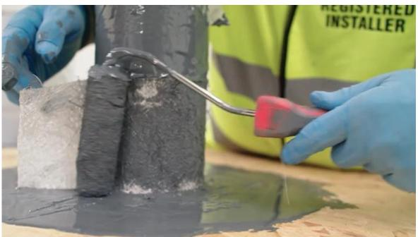
Allow all detail work, including joins, to dry and cure fully before applying the product to the main area.
