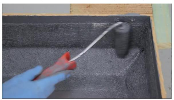
Repeat this process on all relevant areas, considering that joins must be lapped 50mm each side and on any change of material.
