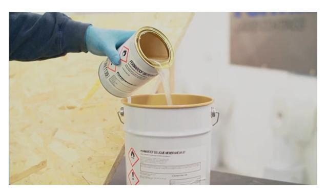
Mix the Permathix into the Permaroof500 (whether accelerated or not) by hand until thoroughly blended. Ensure the Permathix is fully incorporated.
