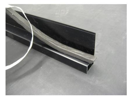
Trim the membrane so that maximum 50mm overhangs the perimeter edges. Starting at one corner, fold the small excess of membrane away...
