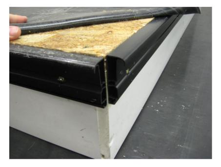
With the membrane hanging over the edges, secure the drip plates. The excess that remains between the two edges can now be covered by a modified Permaroof trim external corner. Remove the excesses as shown below...
