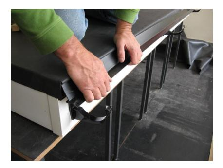
The drip plate can then be tapped firmly into place until it clips in securely. The use of a short piece of batten with a hammer or even a rubber mallet will ensure that the drip plate will not be damaged during fitting. Do not strike the drip plate directly.
