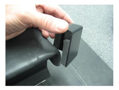
To secure with polytop pins, the corner pieces need to be pre-drilled first for ease of attachment.
