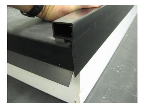
For corner pieces, apply a small amount of Permaroof Bond and Seal or superglue on the inside of the corner, and offer into place. Alternatively, pre-drill a small hole in the side of the corner piece and attach with a poly top pin.
