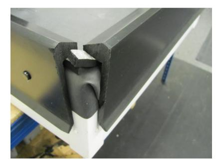
Attach a prefabricated external corner piece and secure with either Permaroof Bond and Seal or Superglue.
