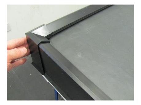
For corner pieces terminating around onto a gutter edge, use a small pre-cut piece of kerb trim and secure with either the sealant or the glue inside the external corner. This will close up the void created by the external corner termination.
