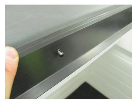
Seal the top edge with an additional bead of Permaroof Bond and Seal, and remove excess sealant.
