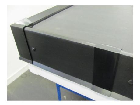
The roof is now ready to receive the Permaroof Plus gutter edge trim drip plate.
