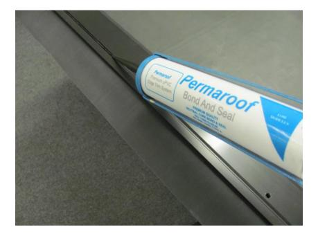
Offer up the drip plate and secure with BP40 polytop pins. Take care not to locate the top of the drip plate higher than roof deck level as this will cause ponding on the roof.
