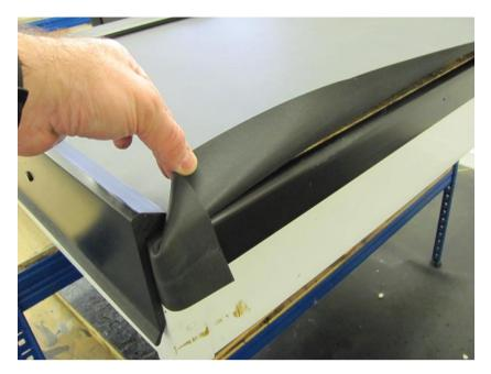
Cut the drip plate to the desired length which will be applied to all existing overhanging roof membrane.
