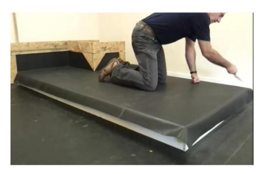
In this example, there are curved edges on the other two dimensions. Trim all edges down to 50 mm.
