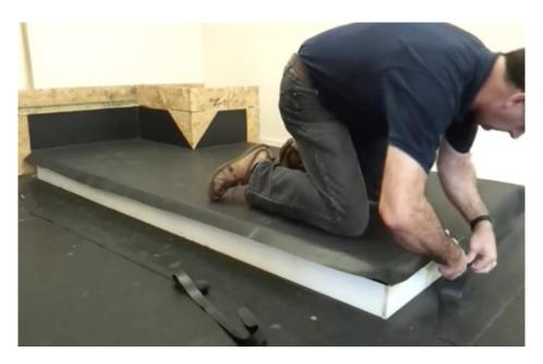
This traps the EPDM membrane between the back plate and the drip plate.
