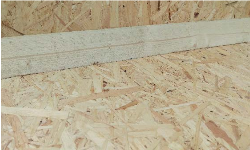
SHOWING UPSTAND WITH TILT FILLET (GRP TRIMS CAN ALSO BE USED):
