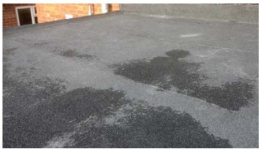
If the felt has been previously overlaid with a liquid coating and has suffered water ingress leading to delamination, remove where possible and again inspect the felt.
