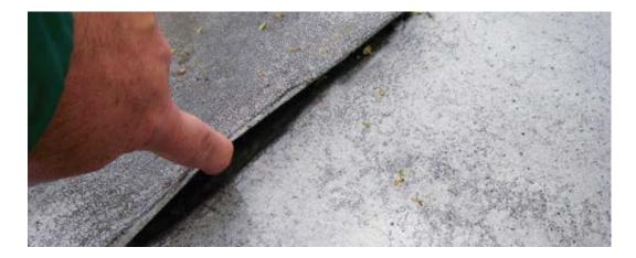
Matting must be used on any joints, cracks or change of materials. Accelerated liquid membrane is applied to the surface, the matting is rolled into the membrane (until liquid membrane is drawn through), then another coat of liquid membrane is applied ensuring the matting is fully embedded.
