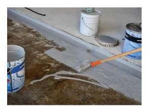
When first opening liquid membrane tins, the product must be stirred thoroughly ensuring any settlement at the bottom is mixed in. Accelerator is then added at the exact ratio of 110ml (of accelerator) per litre of liquid membrane (or 2Ltr/25kg tin or 500ml/6kg tin of liquid membrane) and mixed at a slow speed to avoid air entrapment/bubbles.\*
