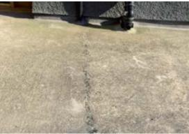
Any small cracks and damaged areas can be repaired with matting embedded in a coat of liquid membrane (AFTER PRIMING). Any significant cracks to be filled using any approved polyurethane based mastic (BEFORE PRIMER IS APPLIED). AVOID the use of silicone based mastics.
