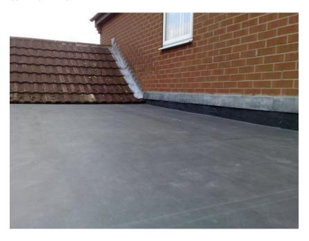
...and also metal wall trim. If attaching metal wall trim into a wall chase, use Permaroof Bond and Seal to waterproof the top edge of this trim, and mechanically fix the trim to the perimeter wall with tech fixings.
