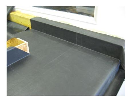
When one wall is completed, repeat the procedure to the adjoining wall. An excess of material will collect in the corner, which needs to be tidied up and secured. This excess is commonly known as the "pig's ear".
