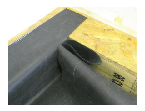
$\ldots$  and the membrane securely adhered.
