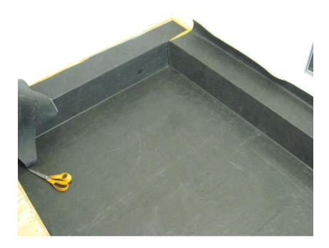
A Quickseam Corner Flashing patch is the finishing detail for this corner...
