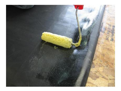
Once the adhesive is tacky, offer up the membrane by rolling it into the angle change and then up the upstand wall. This method prevents any tenting of the membrane at the angle change.
