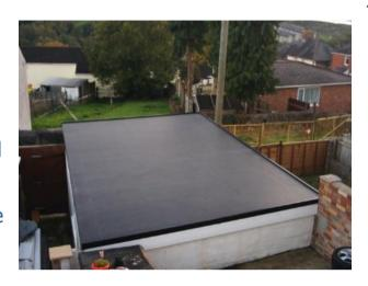
durable, but it may be worth making sure the deck is in good condition before you apply the EPDM membrane. This is because EPDM rubber has an expected lifespan of 50 years or more, and it is wise for homeowners to make sure the deck will last as long.
