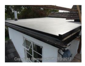
Flat roofs can be installed on anything from a small porch on a residential home, to the large expanse of a commercial building, and will usually have an incline of not more than 10°.
