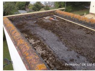
The greatest challenge with flat roofs is their quality and durability. Due to the slight angle of inclination, flat roofs can be a challenge in areas with extreme weather conditions and high humidity. They slow down drainage, creating pools and ice dams, which can cause damage to the roof decks.
