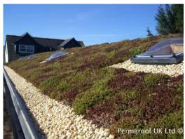
The vegetation may retain a lot of water which may otherwise damage the roof deck or cause leakage, so EPDM can prove to be the ideal waterproofing layer to enhance reliability.
