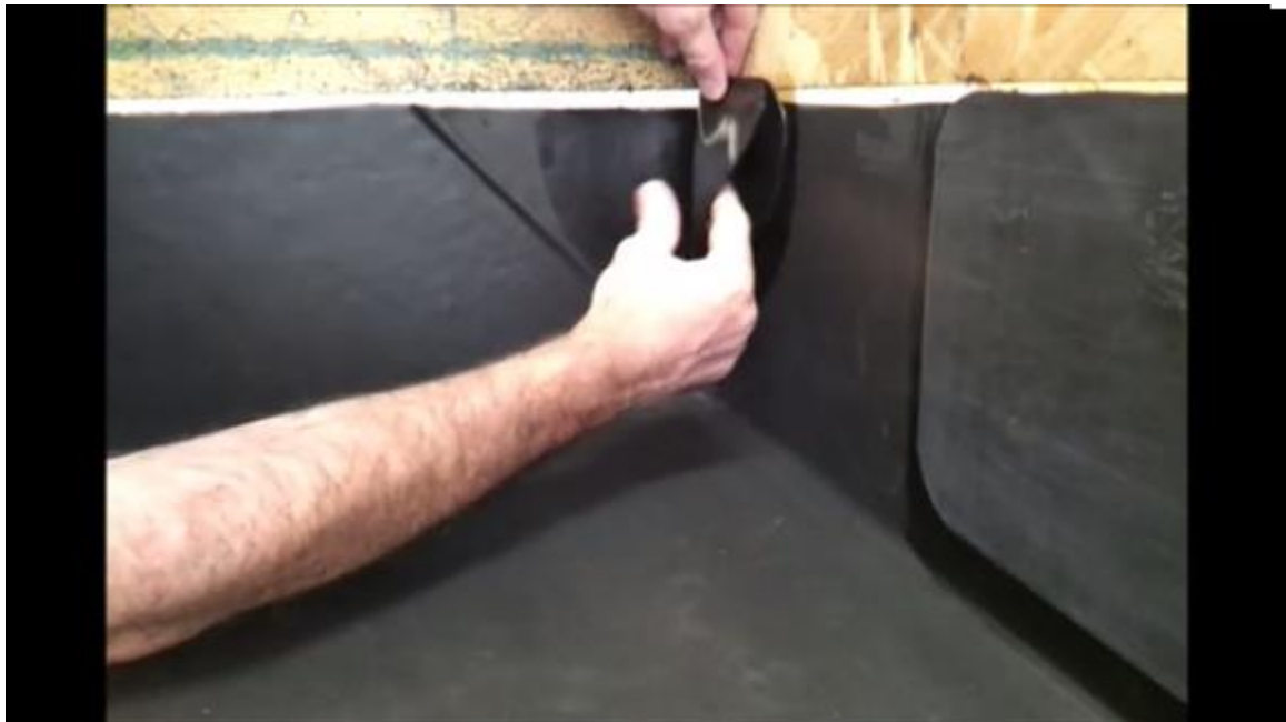
Fig 3: Pressing the FormFlash patch into position.
