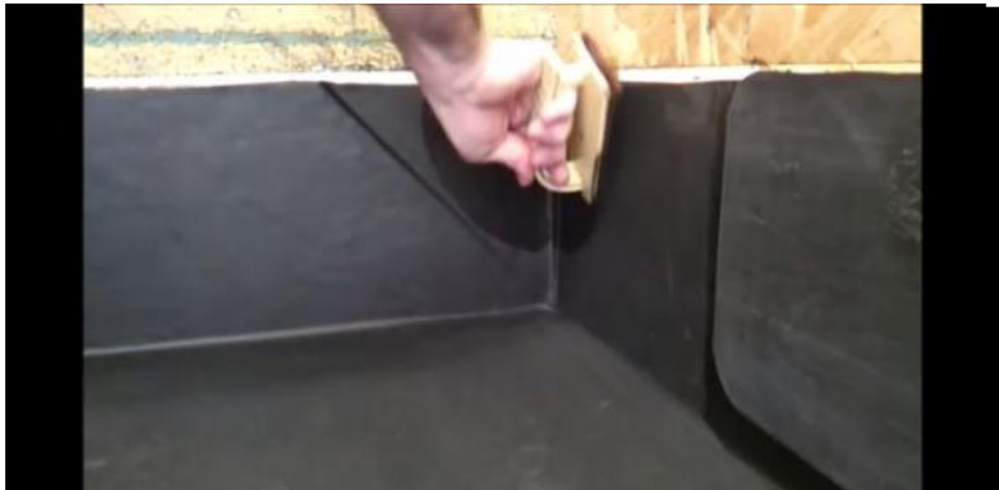
Fig 2: Applying the QuickPrime Plus.
