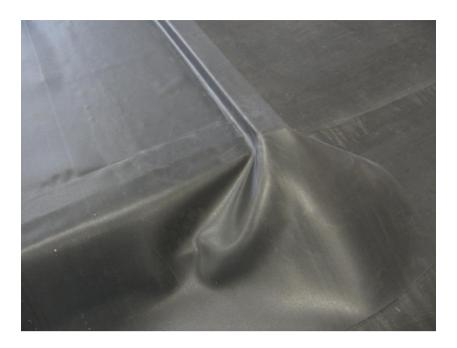
At the gutter edge, excess membrane needs to be trimmed off. Mark the membrane with the blunt edge of the scissors against the gutter (usually 100-150mm from the roof edge) and cut away the excess. The remaining membrane will fall naturally into the gutter at the correct length.
