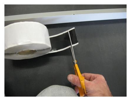
50mm x 25mm of tape is adequate for each fixing. The fixing points are evenly distributed and are generally 600mm apart. Apply the tape to the underside as shown, and peel off the backing paper.
