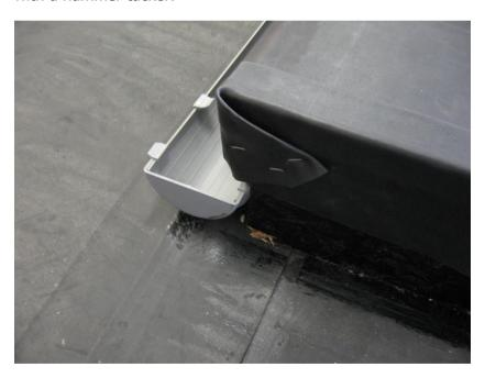
Use the tin snips to cut the trims to size. For corner details, cut the top edge and also a V-shape in the trough at the bottom edge of the trim.
