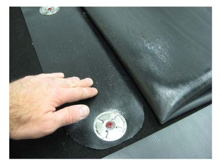
Repeat the procedure on encountering each RUSS strip. Work in one direction e.g. along the width of the roof, then apply the membrane to the strips running down the roof length.
