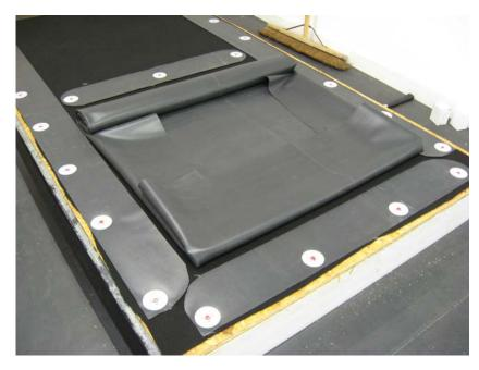
Clean the RUSS and underside of the EPDM sheet with Splice Wash and a cotton rag.
