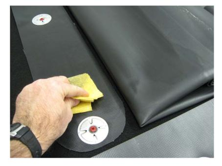
Once the Splice Wash quickly evaporates, Splice Adhesive can then be applied to the same surfaces.
