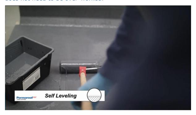
This provides more control over the thickness, which needs to be a minimum of 1.4mm thick, or a coverage rate of 2kg per square metre.
