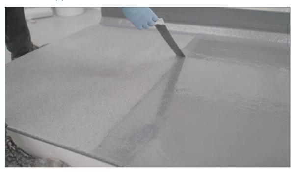
For a finer, encapsulated anti-skid, you can add PermaPlastic to the mixed Top Coat UV at a 10-50% ratio before application.
