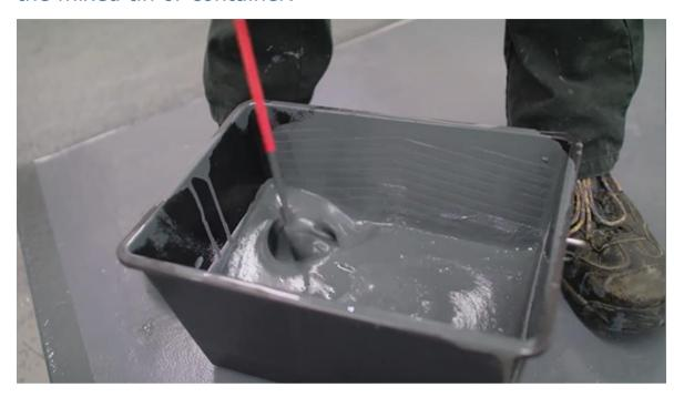
When applying the Permaroof500 Top Coat UV combined with PermaPlastic with a roller, it leaves a finer anti-skid encapsulated in the surface area.
