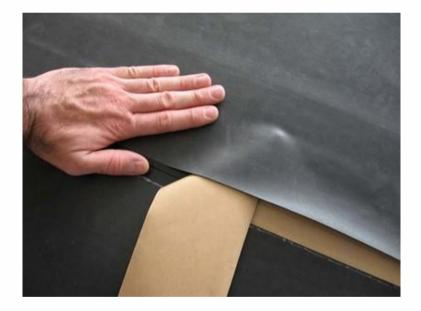
**Step 7:** Lift up the leading edge, and starting from one end of the tape, peel the backing paper towards you, and let the primed leading edge fall onto the tape, flattening down with your hand whilst peeling.
