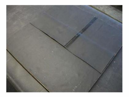
Notes: A T-piece detail is required whenever the end of a seam needs to join an adjacent membrane as shown above.
