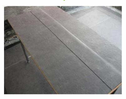
Step 1: Ensure the leading edge overlaps the lower sheet by at least 100mm, and has a straight edge along the entire length of the seam.
