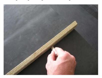
Step 2: Position and mark the sheet with a white crayon. The line should 18mm from the leading edge of the overlap, all the way down the seam. An 18mm timber batten is a useful tool for this.
