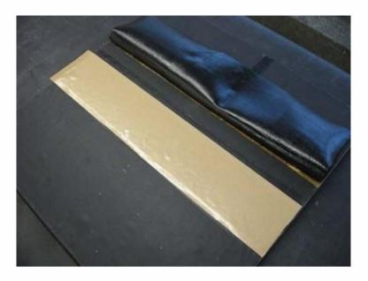
**Step 10:** Do the seam join as usual and use the rollers to firmly press down the seam.
