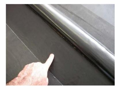
Use the "pushed finger" test, and if the finger moves through the Quickprime Plus or is stringy in any way, it is not ready.
