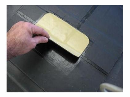
Step 12: Apply the Quickseam Formflash, and use the rollers as normal.
