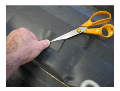
**Step 9:** Cut away the excess membrane as shown.
