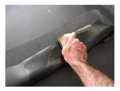
**Step 4:** Apply Quickprime Plus with a scrubber pad and handle, from the marked line and at least 100mm wide. Apply Quickprime Plus to the overlapping membrane also. Apply all the way down the seam avoiding puddles by spreading it out evenly.
