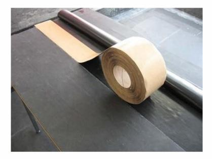
**Step 5:** Once the Quickprime Plus is dry, apply the tape to the primed area. Lay the edge of the roll of tape parallel to the marked line, keeping the tape taut to prevent air bubbles being caught underneath it.
