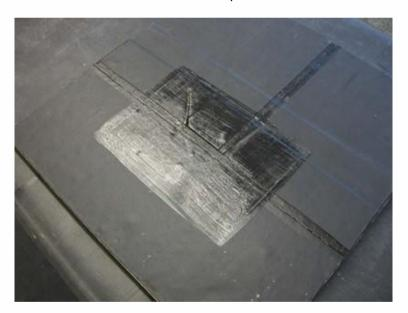
Step 12: Apply Quickprime Plus using the pad, exceeding just beyond the crayon lines.
