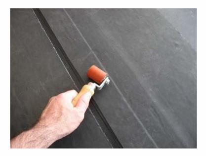
Step 8: Using a silicon hand roller, roll the entire seam thus eliminating any air pockets.
