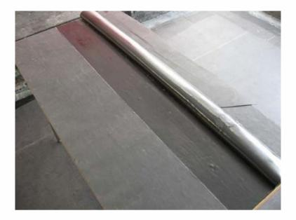
Notes: Wait for the Quickprime Plus to go tacky. This is especially important, as the tape will not adhere to it if it is in a wet state.
