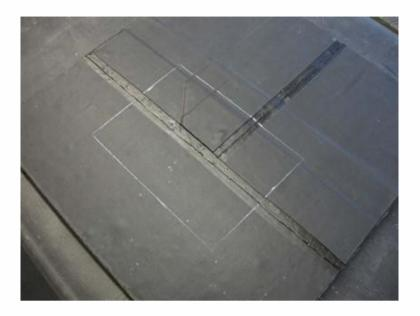
Step 11: This area now needs to be reinforced with a patch of Quickseam Formflash, of size 150mm x 225mm. This covers the necessary 75mm from the weak points. Mark the area to be primed.
