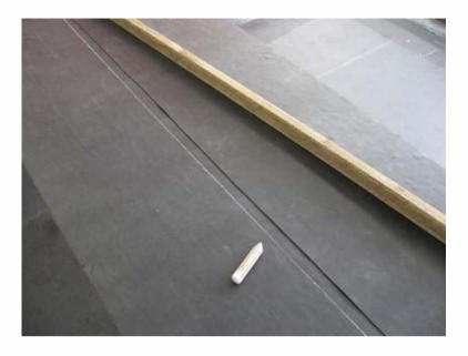
**Step 3:** Flap the leading edge away from the line. It may be necessary to keep it secured with various items so it will not flap back onto your working area.
