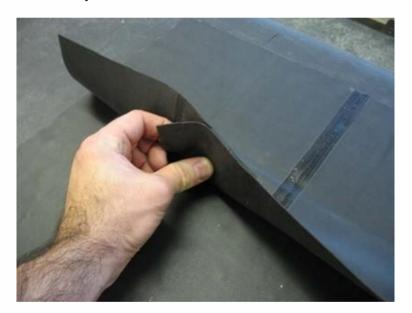
An excess of membrane from underneath the original seam will need to be cut back at a 45° angle. If this is not done, it will leave an unsealed entrance point for water ingress.
