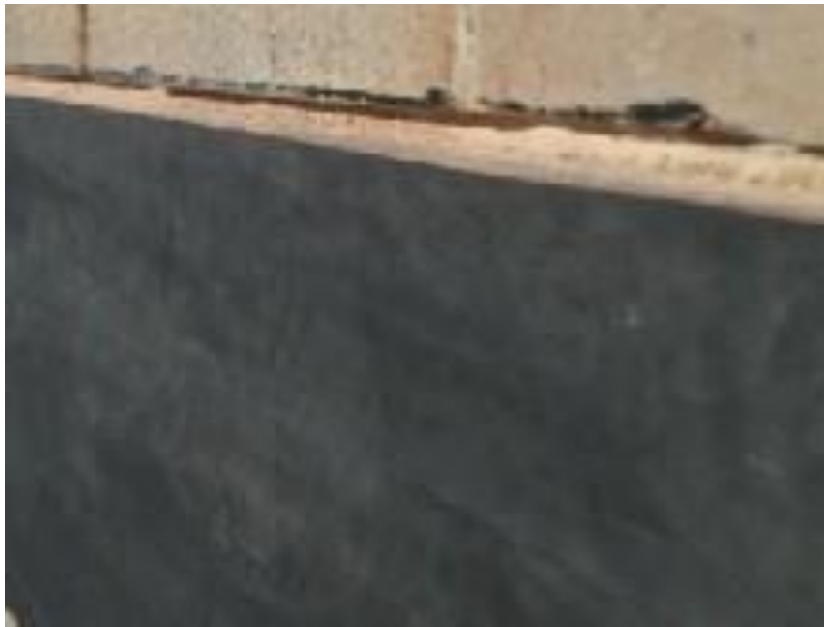
Fig 2: Leaving the EPDM just short of the chase.
