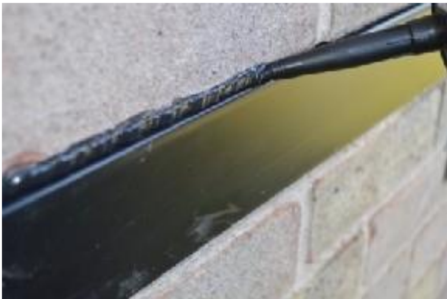
Fig 7: Sealing up the chase with Permaroof Ultrabond.
