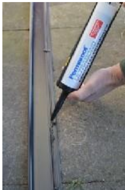
Fig 3: Applying the Permaroof Ultrabond to the reverse of the wall flashing.
