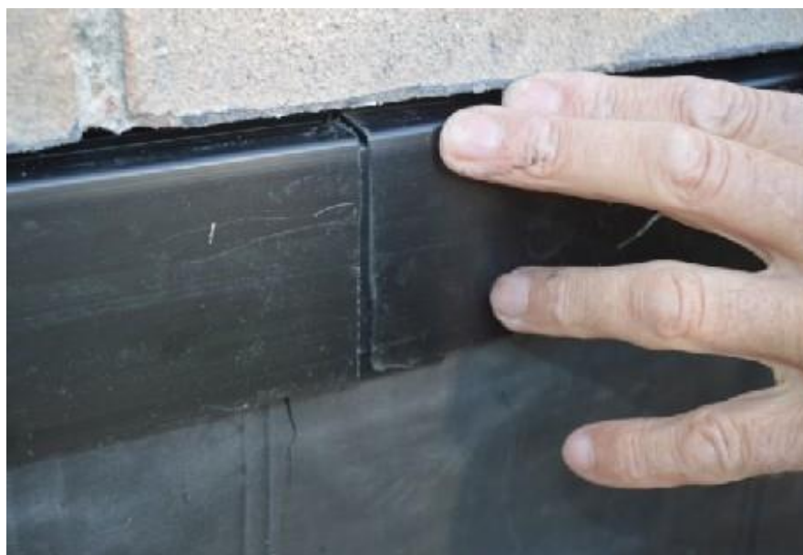
Fig 6: Butt up the next piece of flashing to cover the wall trim.
