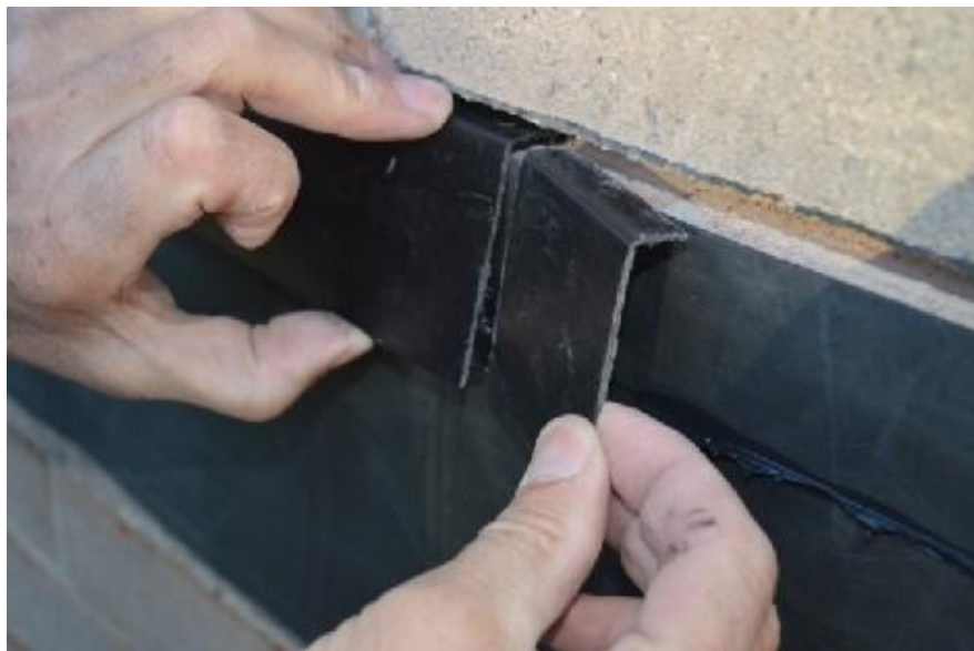
Fig 5: Making a joint clip with wall trim.
