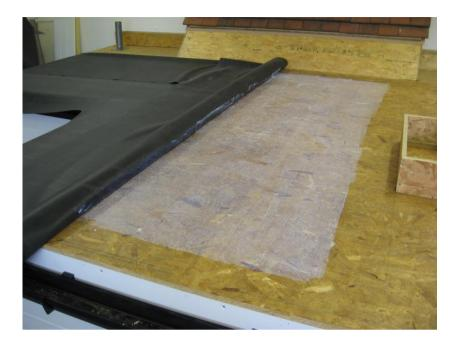
Note that the water-based bonding adhesive does not go right up to the perimeter edge of the roof deck, but instead terminates 100-150mm away. This area is where the Firestone Bonding Adhesive will be applied later. The water-based adhesive can take up to a few hours to grab the membrane completely depending on ambient temperatures, but the use of the Firestone Bonding Adhesive around the perimeter edges secures the sheet in place during this period.
