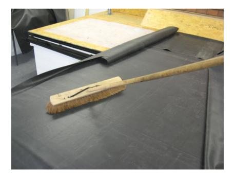
Roll back the other half of the membrane until approximately 100mm of the already applied adhesive is visible and repeat the procedure.
