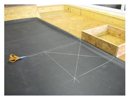
Roll the membrane around the protrusion, leaving a triangle of membrane that turns up all 4 sides.
