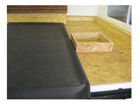
Measure the width and depth of the protrusion and transfer these dimensions onto the folded membrane. Draw an X inside the box.
