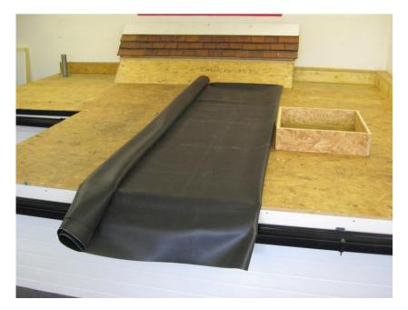
Bonding of the membrane can now begin. Using a 9" roller, apply the water-based bonding adhesive to the timber substrate only.
