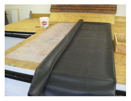
Once the adhesive is applied, the membrane can be laid into it whilst still wet. Roll the membrane into the adhesive avoiding stress or wrinkles, taking care to spot and remove any debris that may have fallen onto the deck in the meantime.
