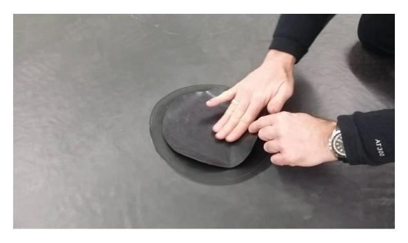
...then go over the top with the silicon roller provided to ensure 100% adhesion.
