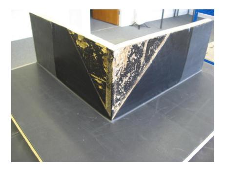
Cut out a piece of SA Flashing and trim the corners.
