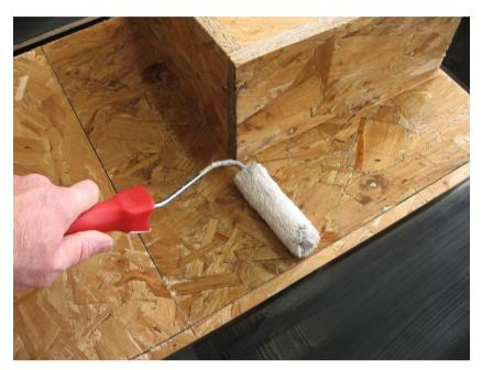
Once the contact adhesive becomes tacky, roll the membrane towards the base of the upstand, pushing right into the angle change to eliminate any tenting.
