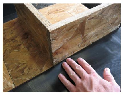
Mark a line with the crayon, at  $45^{\circ}$  from the corner. This will create the resulting V-shape on the upstand.
