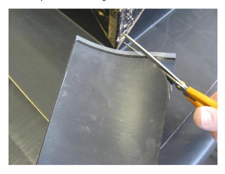
Once the Quickprime Plus is tacky, offer up the SA flashing, using a silicon hand roller to ensure adhesion. Ensure that Quickprime Plus is visible at all edges of the flashing when it is applied. This is less important at the top edge as a metal counterflashing or lead is usually installed here.
