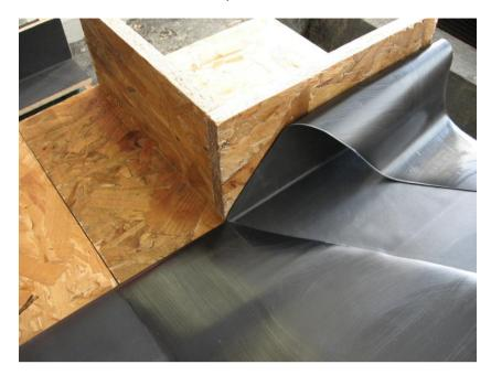
The rest of the membrane can now be applied onto the roof deck around the corner, and then adhered to the upstand using the same procedure.
