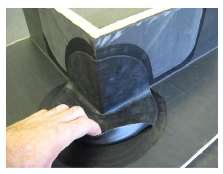
...and use the rollers to ensure adhesion.
