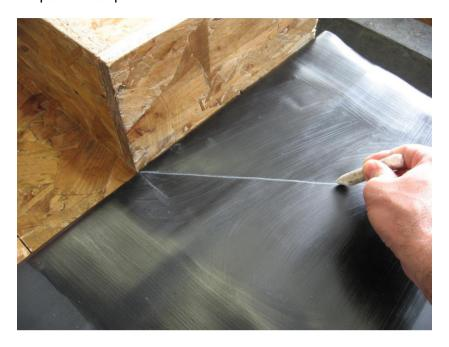
Cut down the marked line until you reach the upstand corner. Also cut away any excess membrane, to make handling the material easier.
