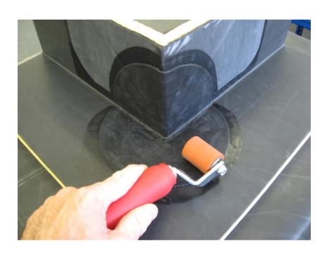
A finished example of a skylight installation using SA flashing and Quickseam corner flashing patches.
