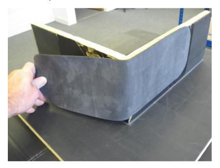
The final waterproofing detail requires a Quickseam corner flashing patch at the corner at the angle change.
