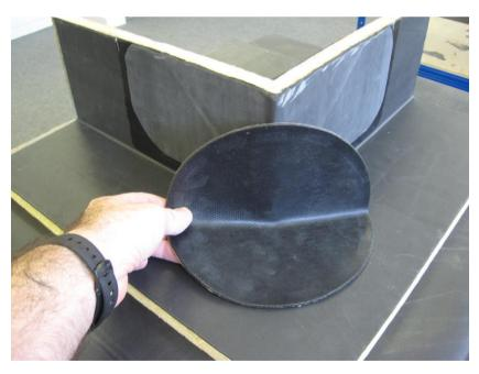
Mark out the area the patch will cover, allowing for a  $25 \mathrm{mm}$  excess and apply Quickprime Plus to this area.
