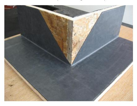
The corner needs to be waterproofed with one piece of SA Flashing and one Quickseam Corner Flashing patch.
