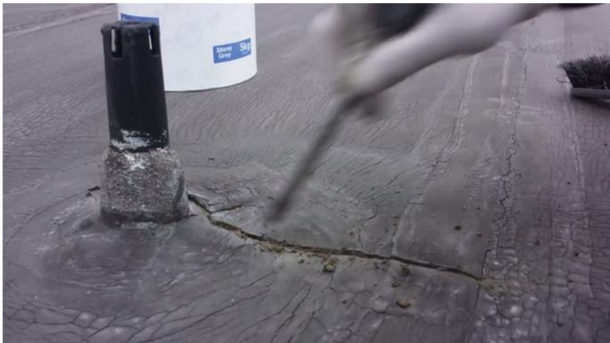
Fig 2 – Clearing the cracks of dirt and debris.
