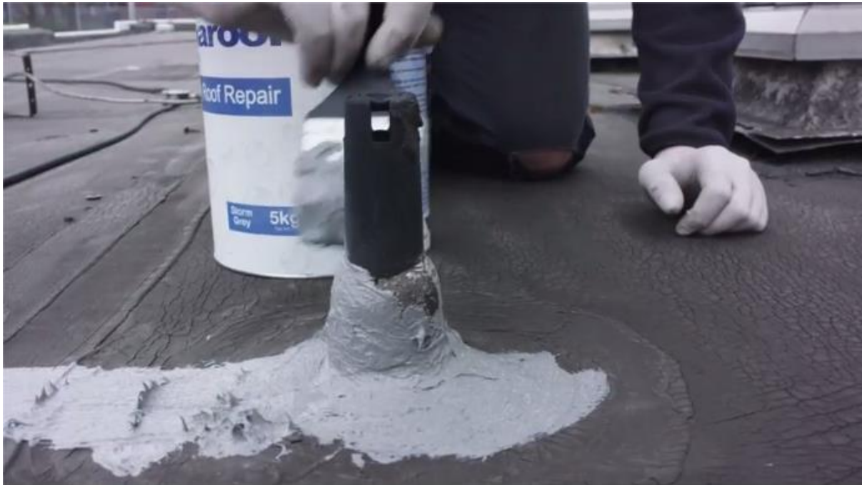
Fig 7 – Applying the product around a pipe extrusion.
