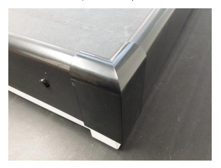
At corners where the kerb edge meets the gutter edge, finish off with the corner end caps. These are attached with a small dab of superglue and offered into place.
