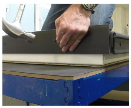
For corner pieces, apply a small amount of Permaroof Bond and Seal or superglue on the inside of the corner, and offer into place.
