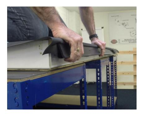
The drip plate can then be attached securely with polytop pins into the pre-drilled holes. Take care not to strike the overhanging EPDM membrane.
