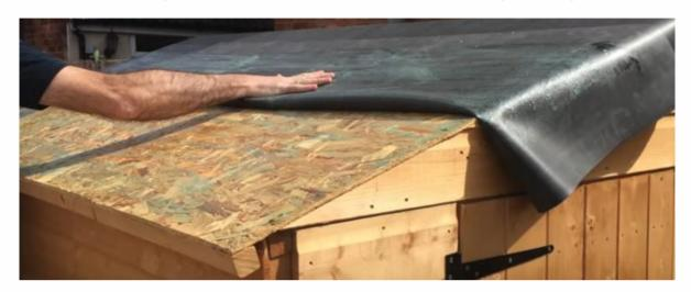
Step 7: Use a soft broom over surface of membrane to ensure full adhesion and to ease out any creases or bubbles.
