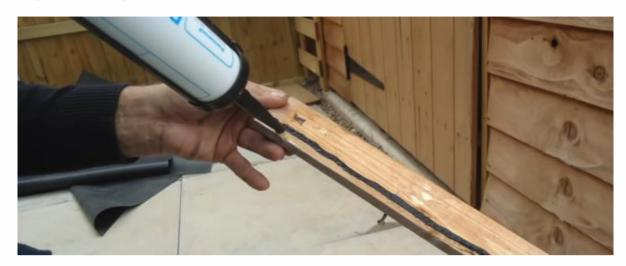
**Step 13:** Sandwich the membrane overhang between the shed and batten. Fix through the membrane into the shed. Ensure the fixing is below the sealant bead for a watertight seal.
