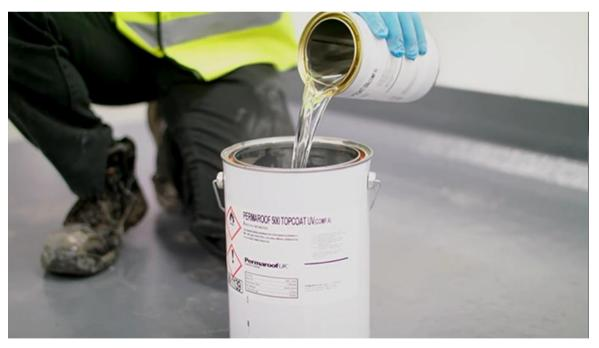
This will cover around 25 square metres, or has a mixing ratio of 6parts A:1part B for smaller areas.
