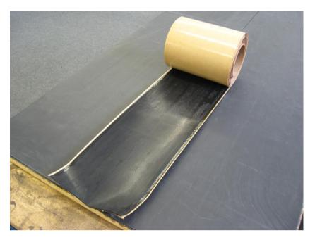
Outline with a crayon where the edges of the tape lie. This gives a guideline for you to apply Quickprime Plus. Make sure that the crayon marks extend beyond the edge of the tape around 20mm each side.
