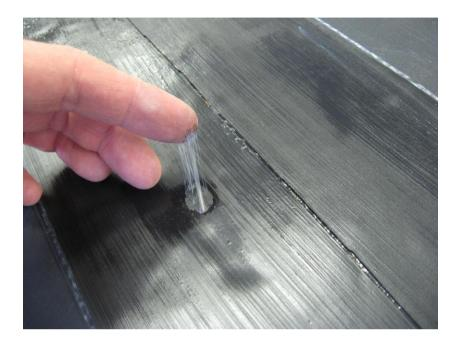
Once the primed surface is ready, apply the tape to the area. Lay the tape parallel to the marked line, keeping the tape taut to prevent air bubbles being caught underneath it. If you run out of tape, overlap the last 50mm with a new roll, but don't forget to apply Quickprime Plus on top of the tape. Continue to lay the new roll of tape. Once the tape is laid, remember to overlay the joint with a 150mm x 229mm patch of Quickseam Formflash.
