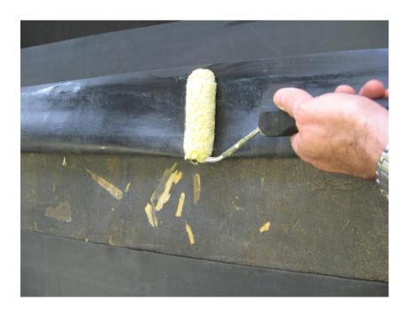
With the membrane now adhered to the deck, lay the tape in situ evenly across the join.
