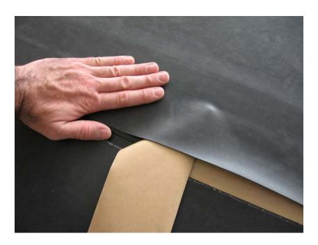
Using a silicon hand roller, roll the entire seam thus eliminating any air pockets.
