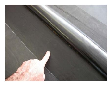
Once the Quickprime Plus is dry, apply the tape to the primed area. Lay the edge of the roll of tape parallel to the marked line, keeping the tape taut to prevent air bubbles being caught underneath it. When applied, if the tape veers off at an angle, cut it, peel the backing paper and overlap the tape by at least 50mm. Continue to lay the tape. This ensures you stick to the marked line. This also applies if you run out of tape, and have to start a new roll.
