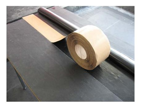
Use the silicon roller to ensure the tape has adhered properly to the membrane.
