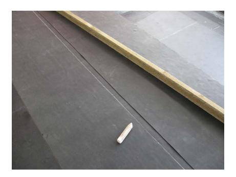
Flap the leading edge away from the line. It may be necessary to keep it secured with various items so it will not flap back onto your working area. Apply Quickprime Plus with a scrubber pad and handle, from the marked line and at least 100mm wide. Apply Quickprime Plus to the overlapping membrane also. Apply all the way down the seam avoiding puddles by spreading it out evenly.
