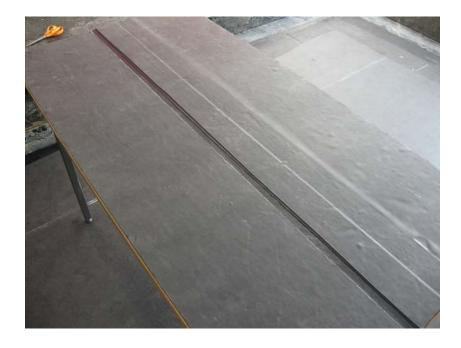
A T-piece detail is required whenever the end of a seam needs to join an adjacent membrane as shown below:-
